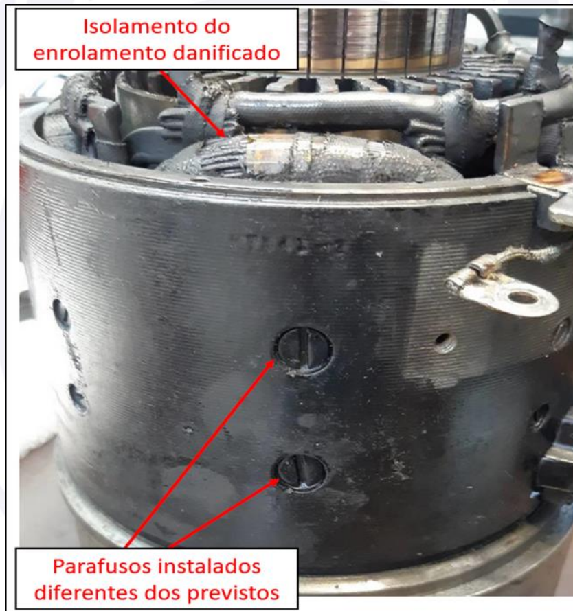
Figure 24 - Evident non-conformities in the casing and winding of the Starter-Generator .
